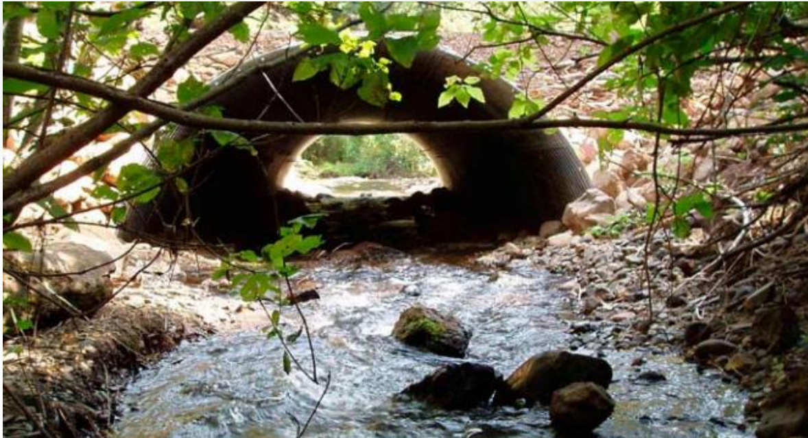
Fish passage culvert
